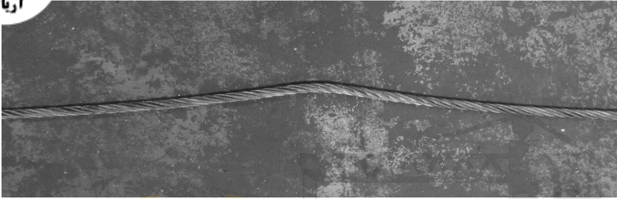
Figure 30-1.8.2-2 Distortion of Rope Structure — Dogleg
