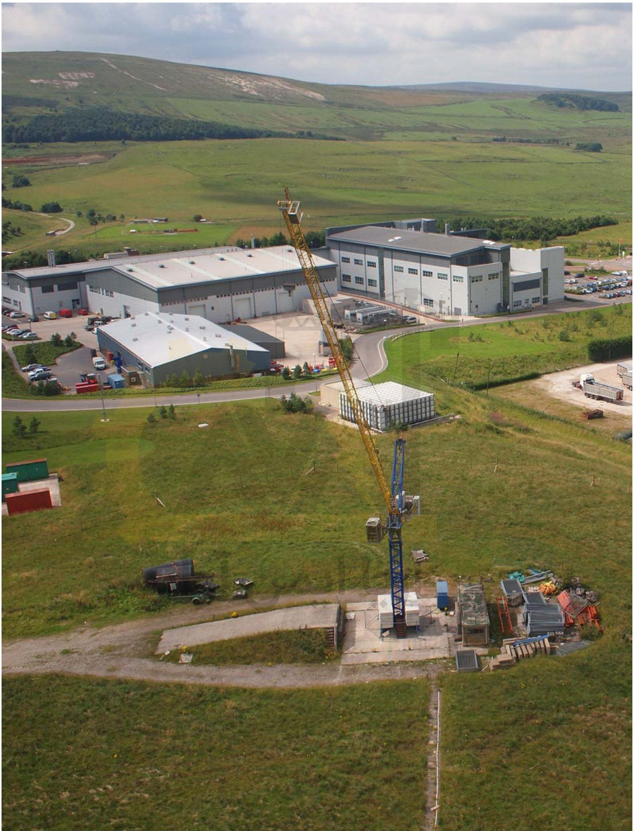
Figure 2 – General View of the Crane erected at HSL HSL VPS Photograph 1004014_058.jpg (cropped)
