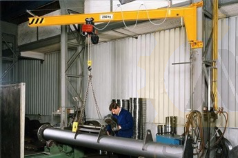
Wall mounted crane
